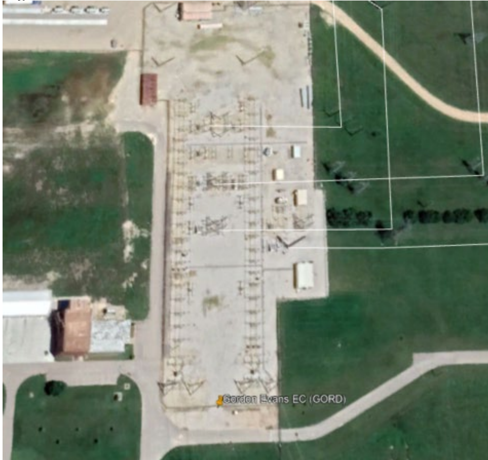
Figure 33 – Gordon Evans 138kV Substation
